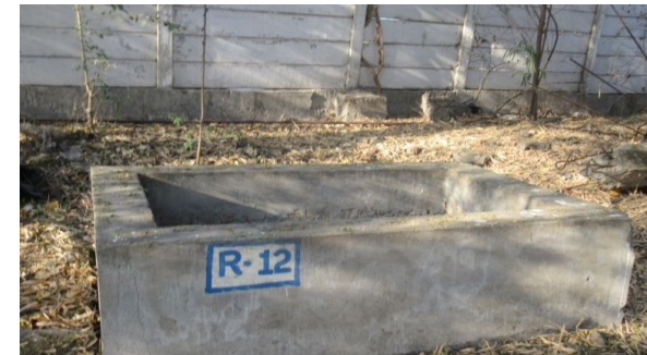
Recharging Pit- 12 Near AAQMS station
