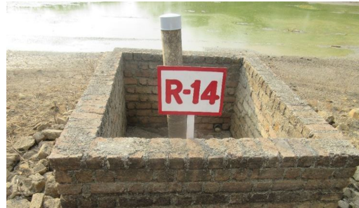
Recharging Pit- 14 In Rain Water Harvesting Pond
