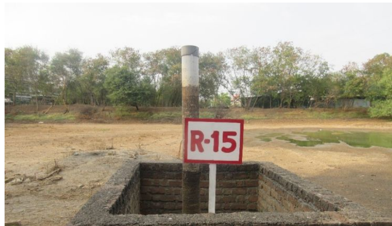
Recharging Pit- 15 In Rain Water Harvesting Pond
