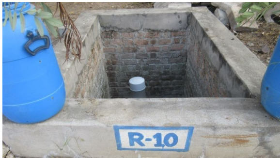
Recharging Pit- 10 Near AAQMS station
