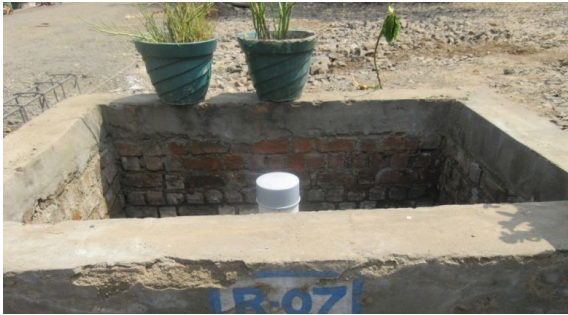
Recharging Pit- 07 Near IBD- XXII
