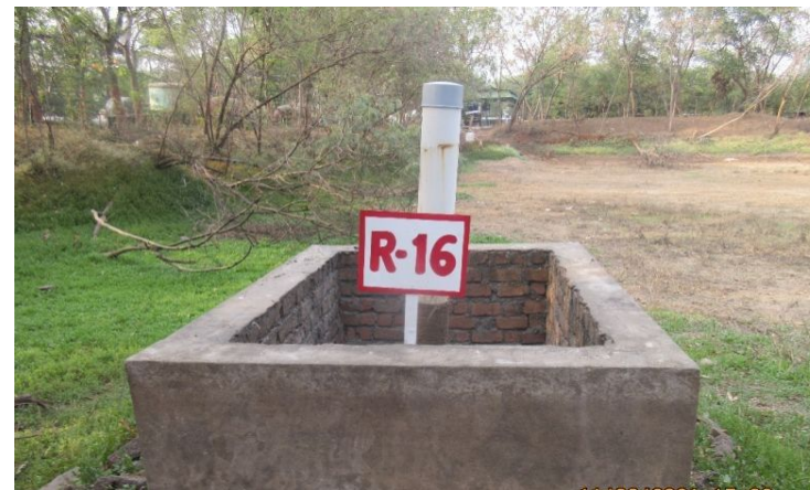
Recharging Pit- 16 In Rain Water Harvesting Pond
