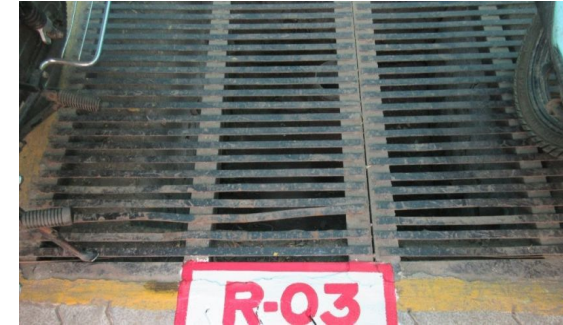
Recharging Pit- 03 Near Gate No. 03
