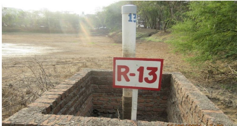
Recharging Pit- 13 In Rain Water Harvesting Pond
