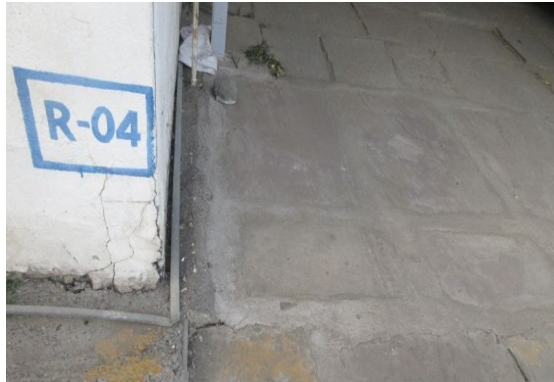
Recharging Pit- 04 Near Gate -03 (A) Car parking area
